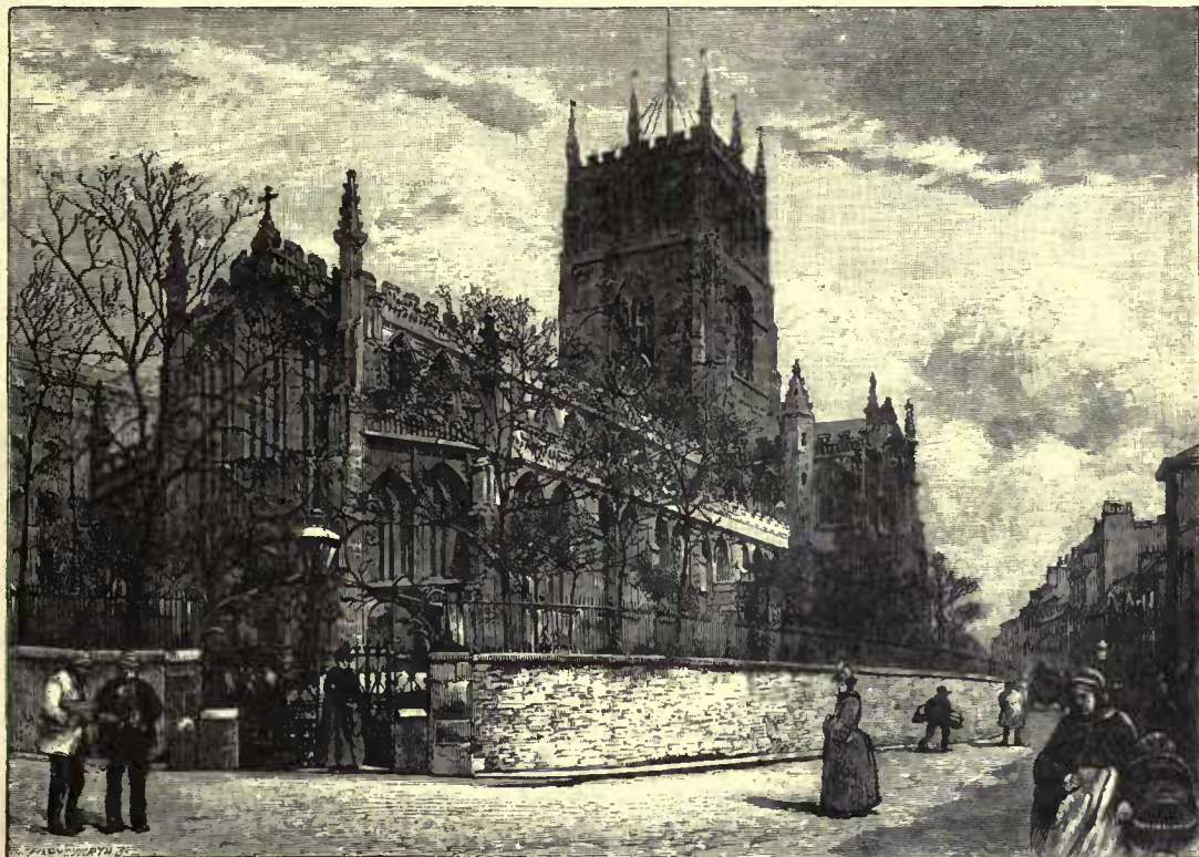
ST. MARY'S CHURCH, NOTTINGHAM. (From a Photograph by Frith & Co.)
